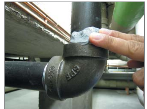
Stop leaks on cast iron pipes
