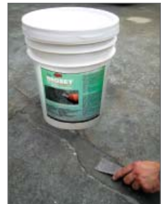
Concrete floor repairs
