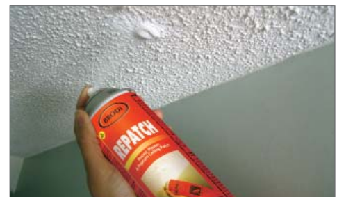
Repairing stucco ceiling
