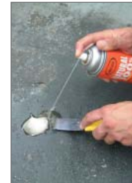
Cleaning grease and grime off concrete floor
