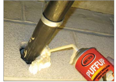
Sealing gap around piping
